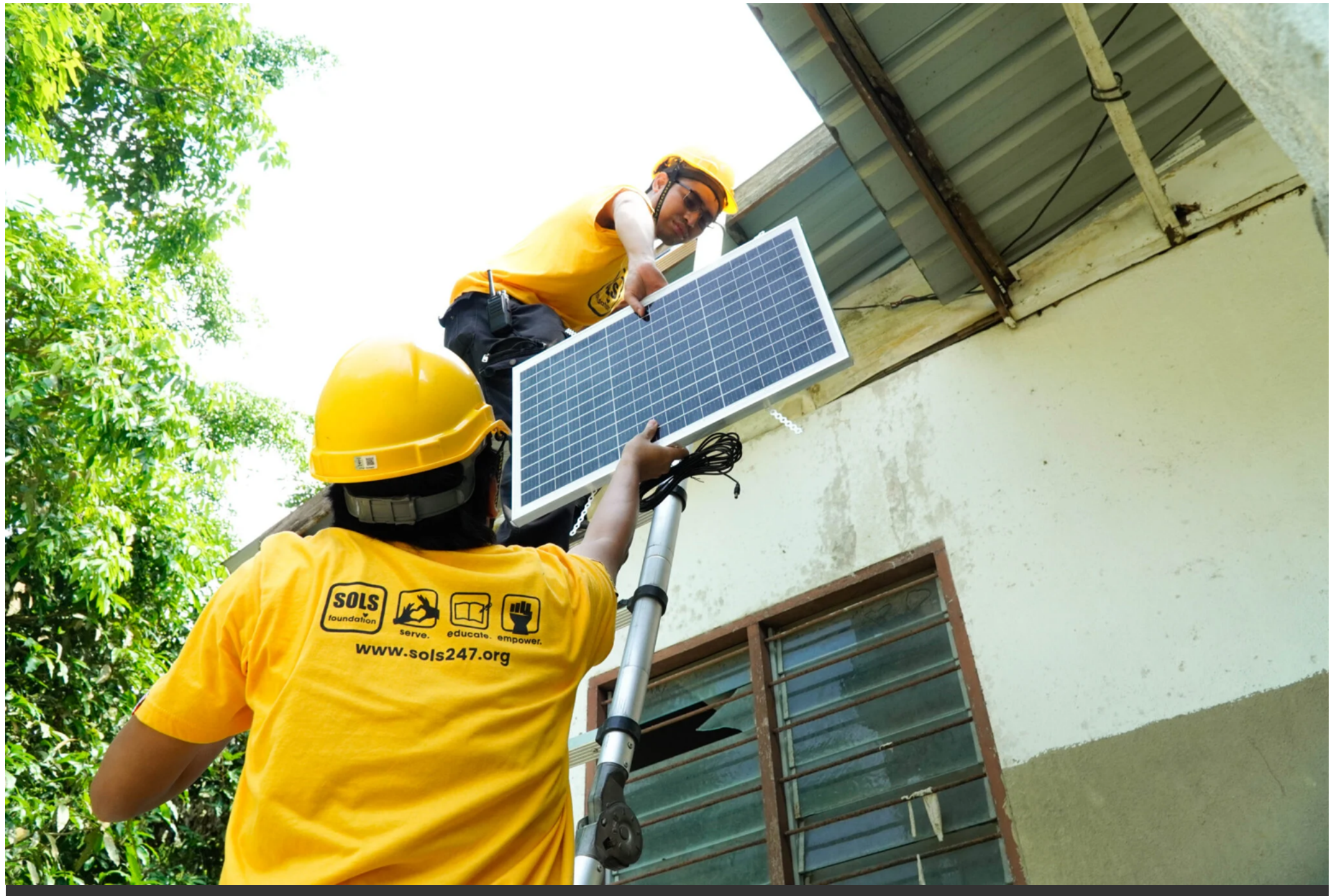
SOLS Foundation team members install a solar panel at one of the 11 participating households in Kampung Sungai Relang.
