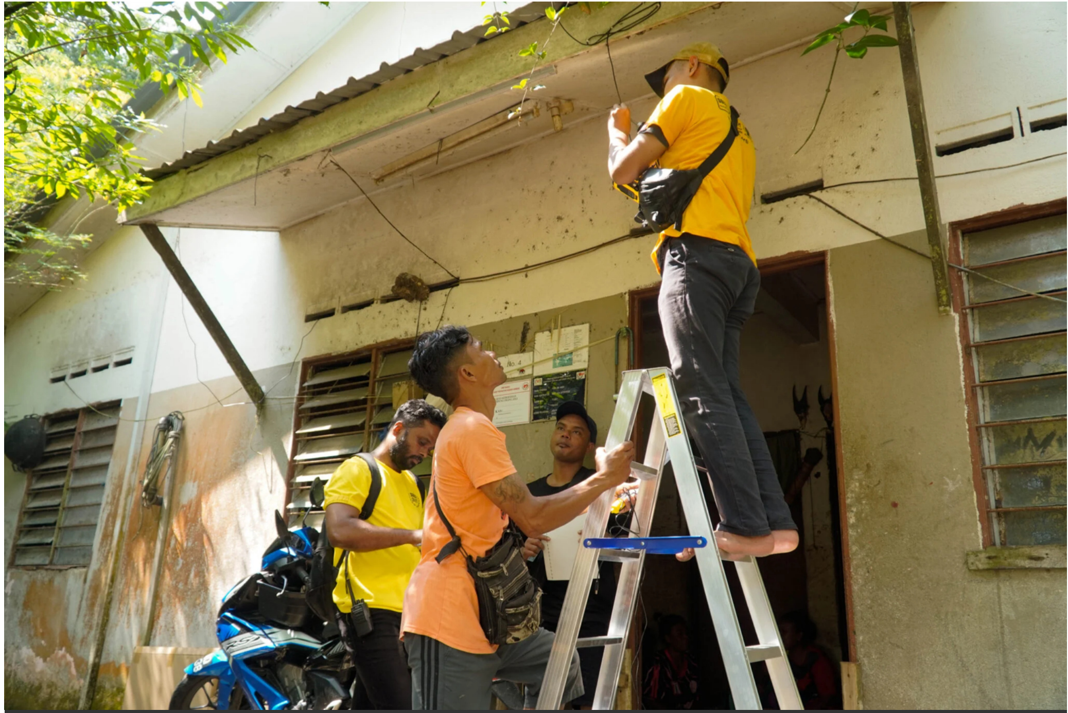
The deployment team completes electrical wiring at a participating household. SOLS Foundation provided the technical expertise for the installation, while volunteers from Google supported the team throughout the hands-on deployment.
