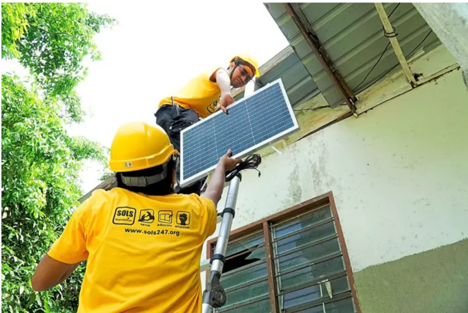
SOLS Foundation team members installing a solar panel at one of the 11 participating households in Kampung Sungai Relang in Hulu Gombak, Selangor, — Handout
